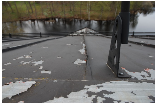
Norra takfallet innan rengöring.
