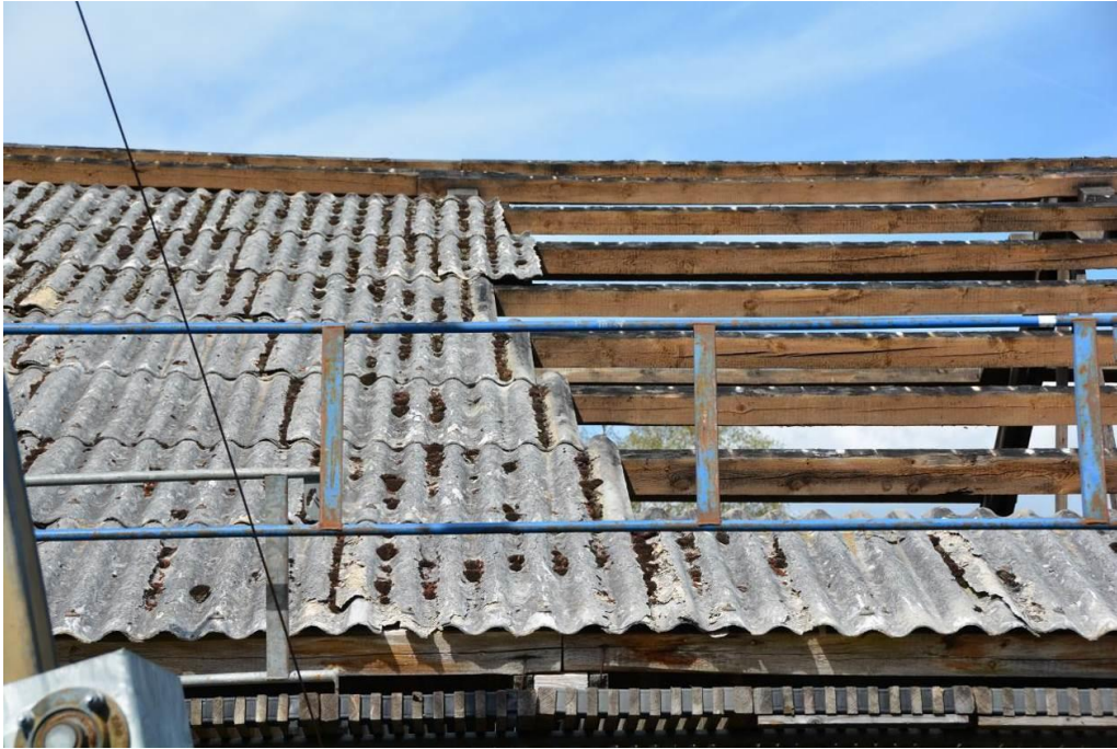
Asbetsplattor under nedmontering. Vlm_kmvVB-588
