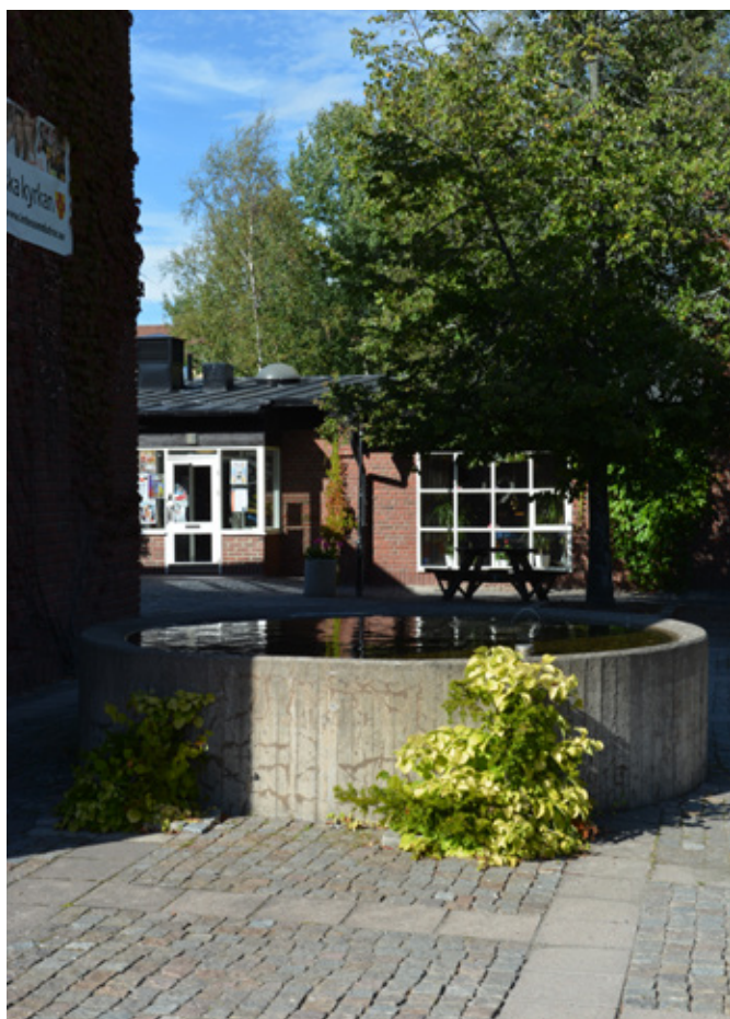
Springbrunn gjuten i betong. Vlm_modkaEK-2874.
